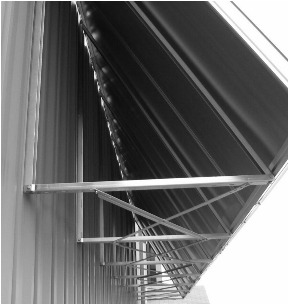
Figure 5.4.5: Typical wall-mount installation of a 60° collector array.
